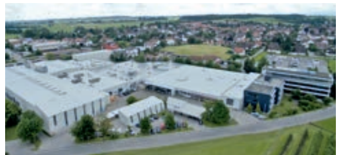
mayr ®-headquarters in Mauerstetten
