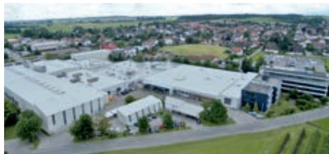
mayr ® headquarters in Mauerstetten
