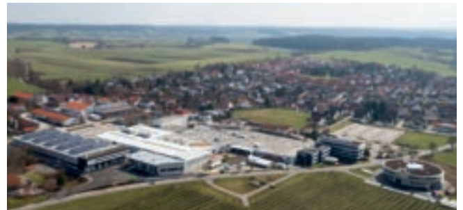
mayr ® headquarters in Mauerstetten: Climate-neutral since 2020
