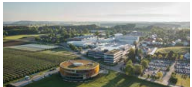
mayr ® headquarters in Mauerstetten: Climate-neutral since 2020
